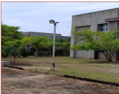
Fig 10: Photograph of LED Street light
