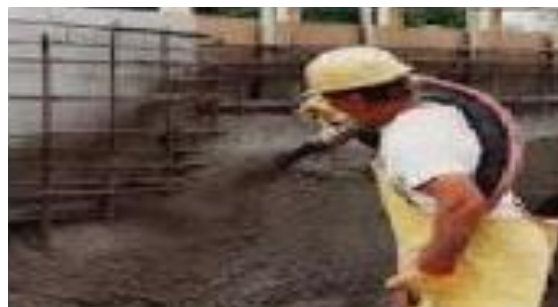
Figure 13: Ferrocement technique
