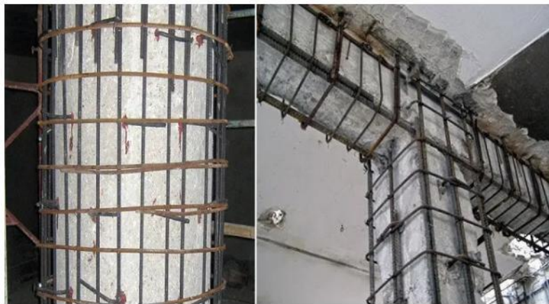
Figure 11: Concrete column beams strengthening
