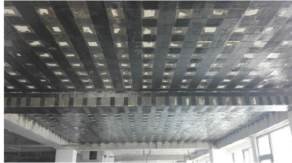
Figure 8: Strengthening by fibre reinforced polymer
