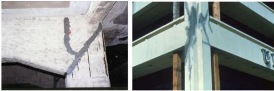
Figure 14: Application of the epoxy resin & cement grout injection in beam–column joint
